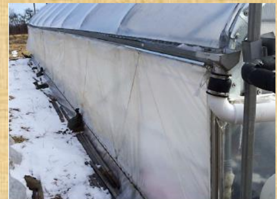
Some high tunnel manufacturers offer substantial gutter systems to collect water for irrigation. Photo: Chris Lent, NCAT
