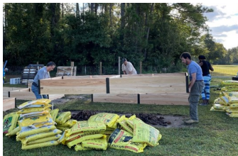
Raised garden beds construction, photo: C. Balliet
